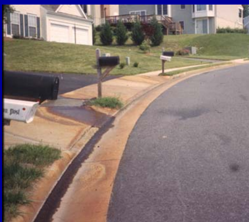
Iron-staining along curbs and sidewalks through the Hampton Oaks subdivision. Homeowners in this neighborhood apply the equivalent of 2 Mg agricultural lime per ha per month to maintain soil pH above 5.5.
