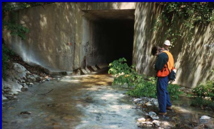
Culvert beneath I-64 in Clifton Forge
