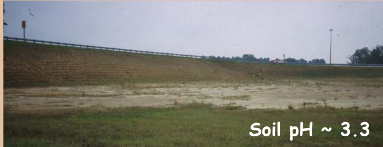
Roadcut along 64E in Suffolk.
