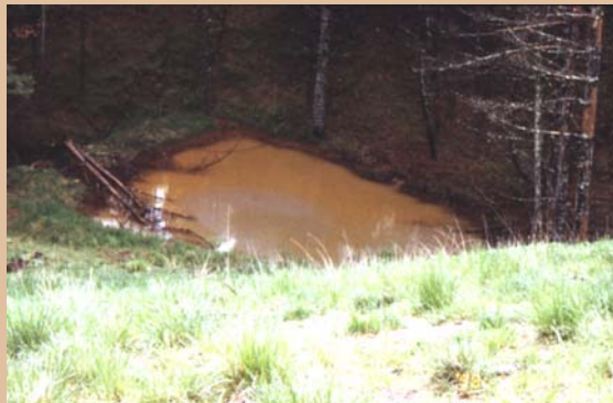
The Rt-250 roadcut drains to this sedimentation pond.
