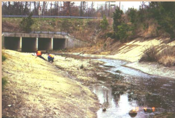
Chesterfield County: Proctor's Creek was redirected to this excavated channel during road construction.
