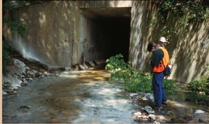
Culvert beneath I-64 in Clifton Forge
