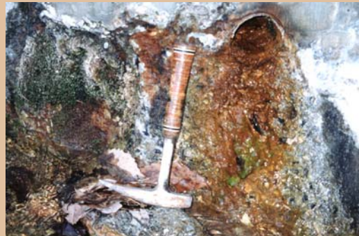
Inside the culvert at Clifton Forge.
