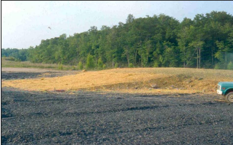
**Topsoil thickness trials being installed in Wise Co. Soil cover was varied from 0 to 1 m with and without 25 Mg/ha lime at contact.**
